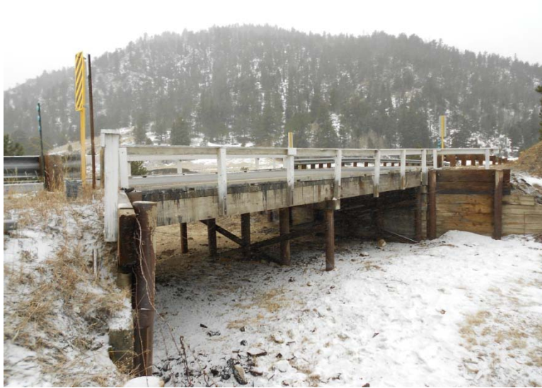
View of Bridge Structure ID: J-14-C on State Highway 9.
